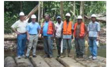
From left Mr. Evans, Mr. Cresson, FTCI Staff and MACORP representative on the bridge being constructed by FTCI
